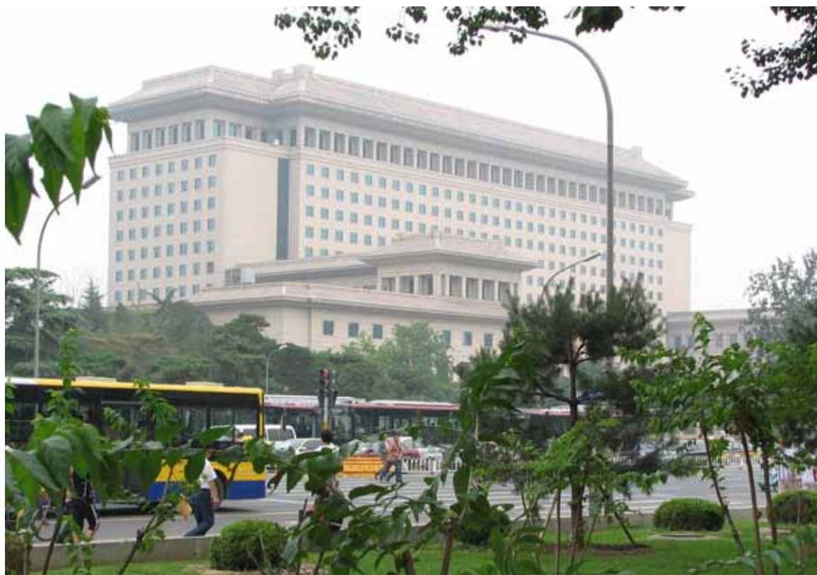
Fig. 1.20. August First Building (Military Commission Headquarters), 1999. Zhang Qiming and others. Photograph by author.
