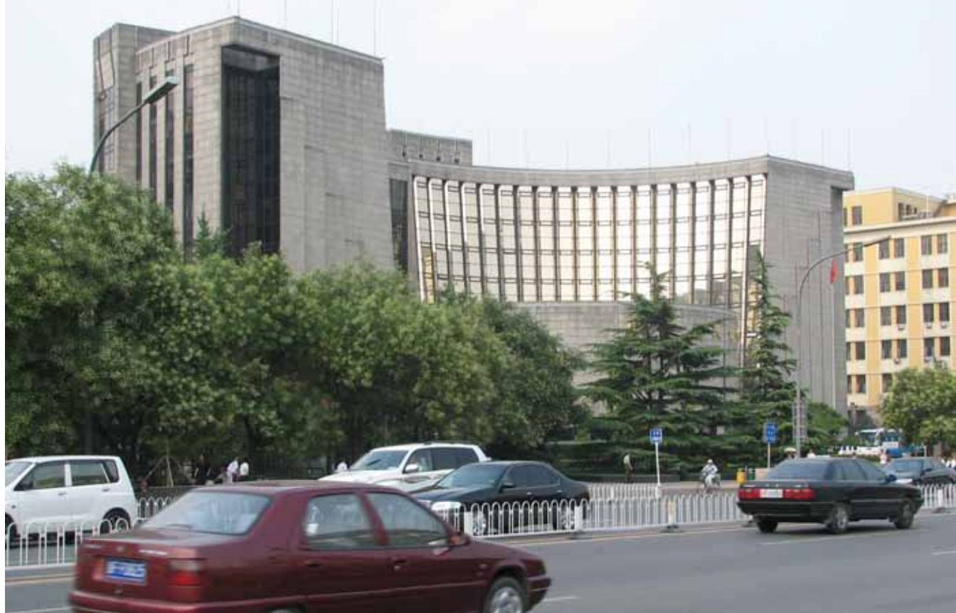
Fig. 1.17. Headquarters of People's Bank of China, 1987–90. Zhou Ru and others. Photograph by author.
